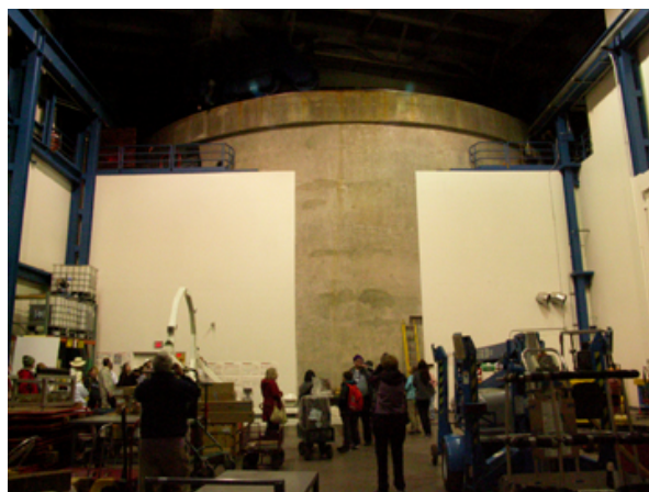
The massive pier of the LBT, 42 feet in diameter.
